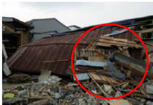
Figure 3. Wooden house structures that are easily destroyed and washed away by a tsunami.
