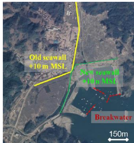
Figure 2. Seawall in Taro City Source: (Uppasri et al., 2013)
